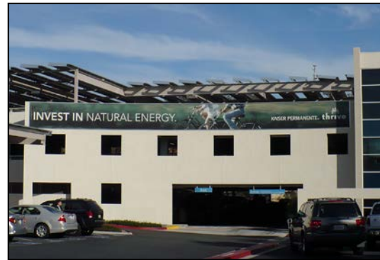
Solar panels line the roof of the parking garage at the Kaiser Permanente Campus.
