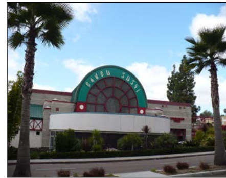
Restaurants replaced a former movie theater on Fletcher Parkway.
